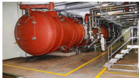
Existing facility for extraction/dry
