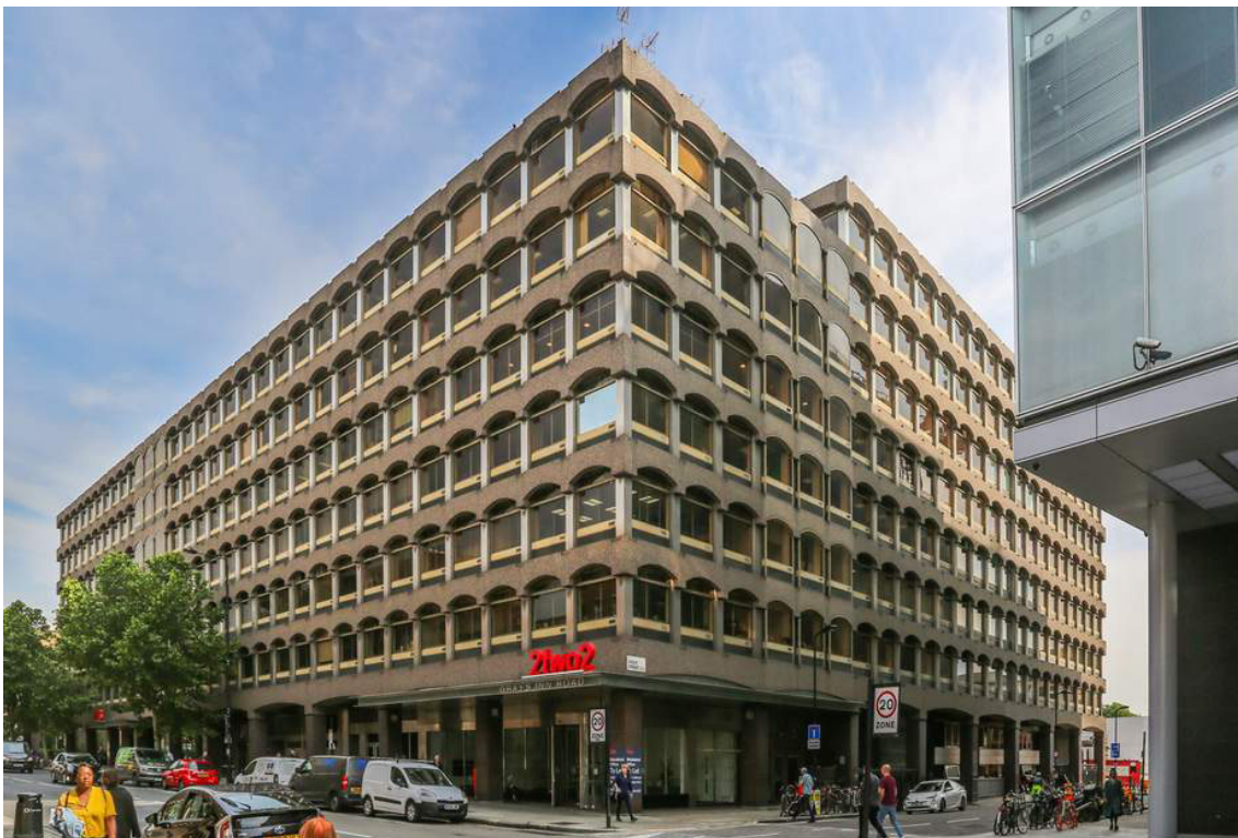
ICO Headquarters is located on the 4th floor of 222 Gray's Inn Road, London
